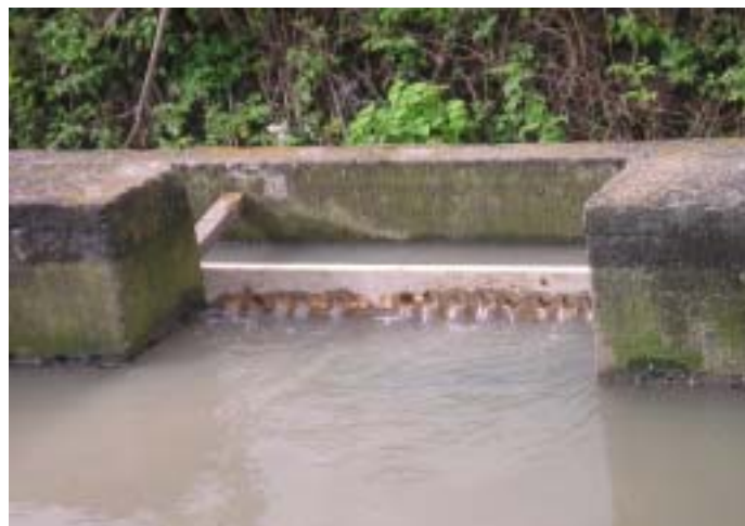
Figure 5.15 Inlet Baffles
