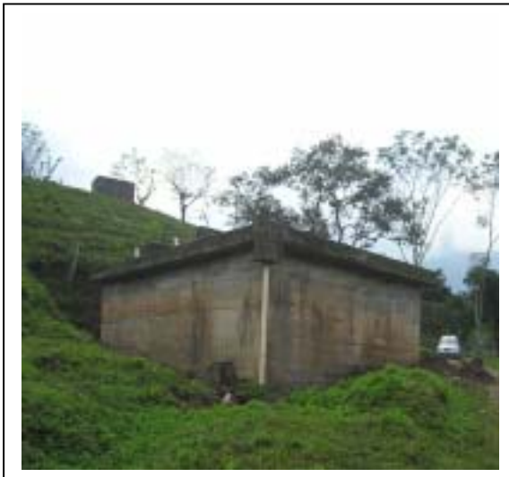
Figure 5.3 Las Vegas Imhoff Tanks
