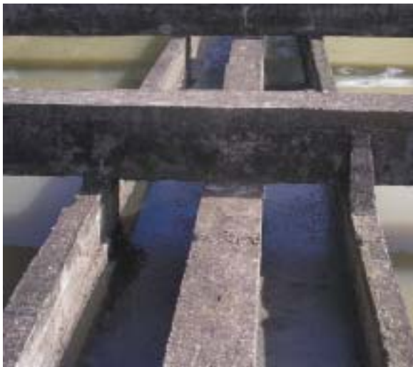
Figure 5.16 Inner Scum Chambers
