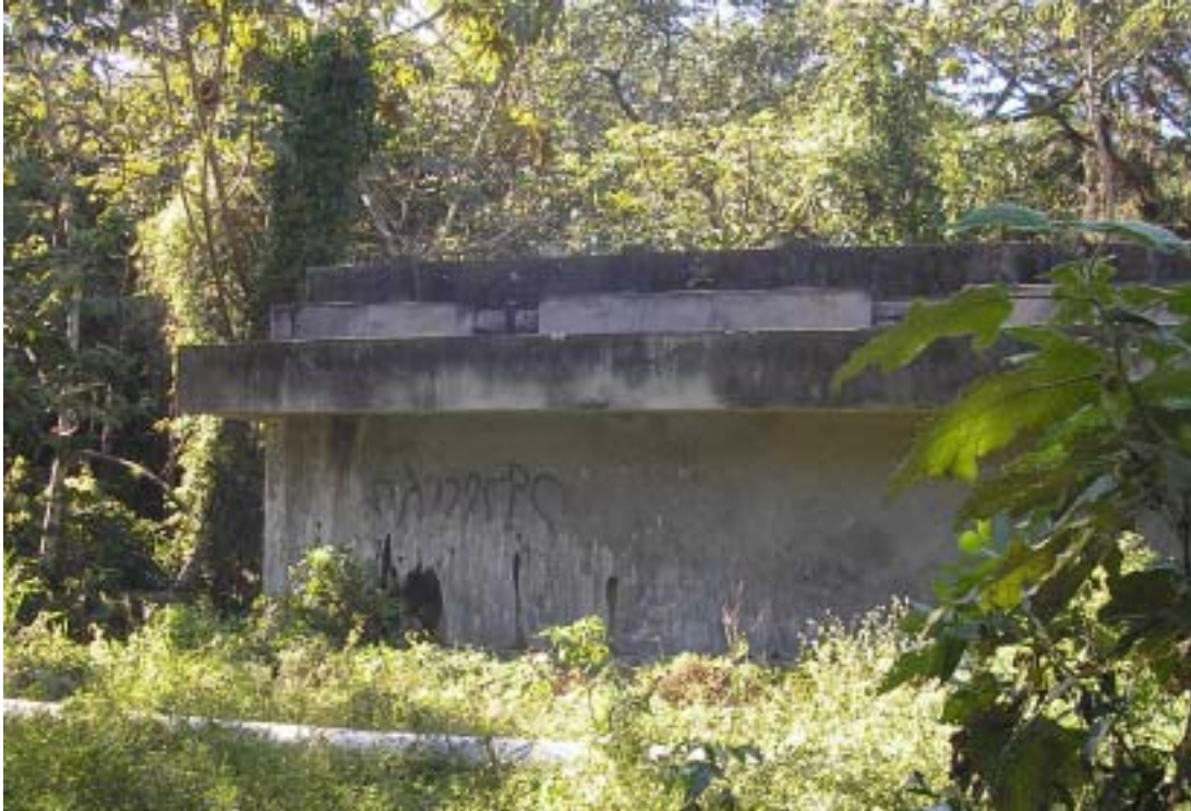
Figure 7.5 Barrio Galeras Imhoff tank
