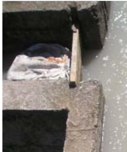
Figure 5.14 Wooden + Sand Bag Flow Gate
