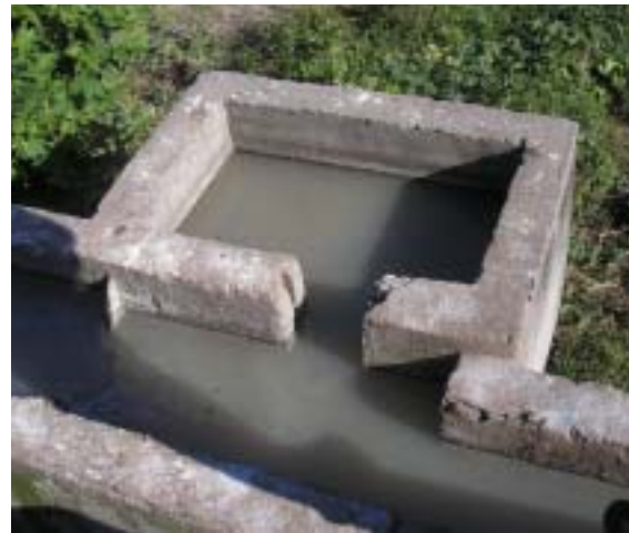
Figure 7.7 Barrio Galeras Bypass
