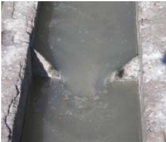
Figure 7.6 Barrio Galeras V- Notch Weir
